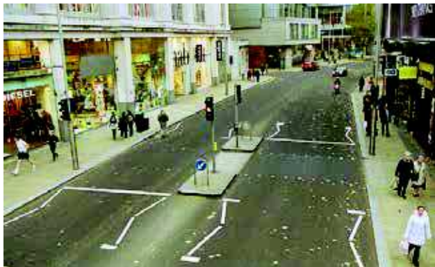
Figure 38. | Even on busy roads zig-zag road markings do not need to exceed 2 on both sides. Kensington High Street
