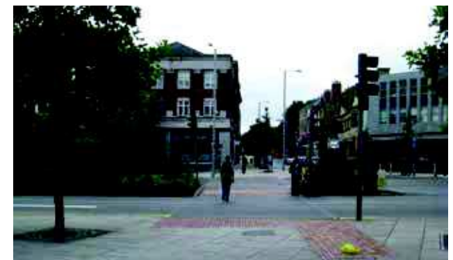
Figure 93. | Maid Marion Way, Nottingham, improvements: formerly a dual carriageway roundabout with underpasses for pedestrians, made into a surface signalised crossing without detriment to through traffic
