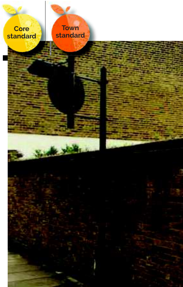
Figure 34. | all signs, lamp columns, sign posts and sign backings, lights and fittings in Core and Town Standard areas to be painted Raven 18B29
