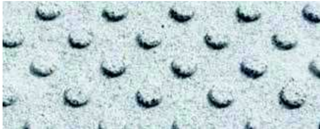
Figure 25. | Core standard tactile paving shall be silver grey ground granite blister slabs with flat top blisters shaped to DfT Guidance
