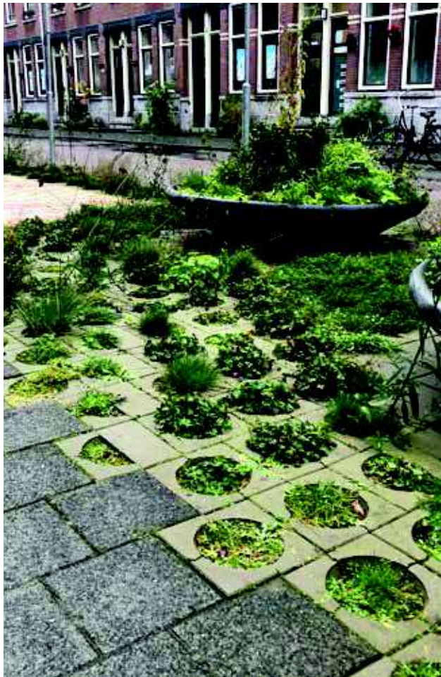
Figure 70. | Above and above right. Planting in footway spaces to encourage water infiltration - Rotterdam (paving specials www.struykverwoinfra.nl/ )
