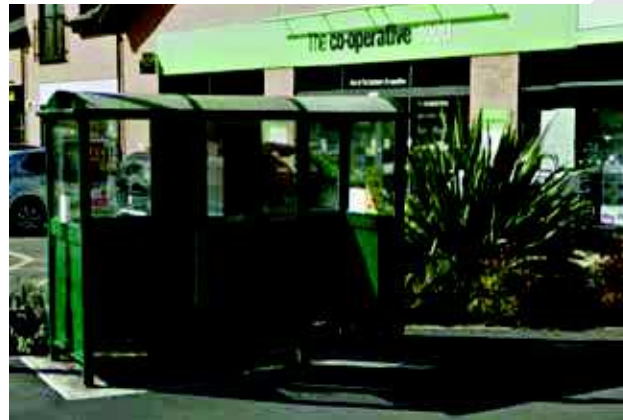
Figure 52. | Many bus shelters are uninviting and poor quality- their second class nature discourages use and can lead to loss of service routes as a result of low ridership. This type will no longer be used within Taunton Garden Town.
