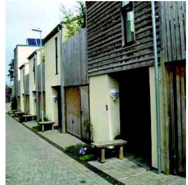
Figure 55. | In housing developments a privacy strip behind the footway or shared surface can be occupied with seats and planting (Ikon, Street)
