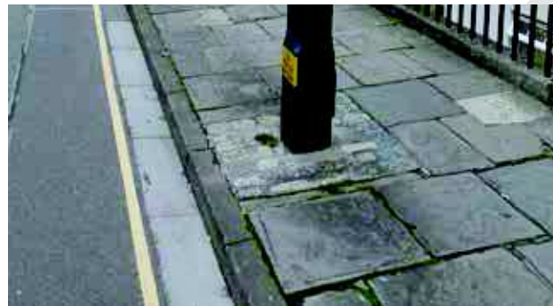
Figure 31. | Yellow lines will be 50mm Primrose everywhere in the town centre beyond the Restricted Zone to reduce visual impact (note: Restricted Zone has no yellow lines)
